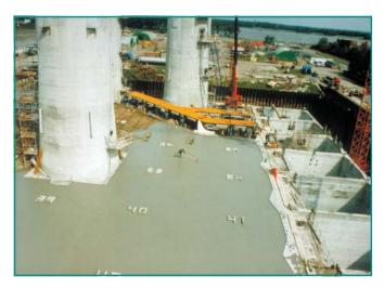
Large number were set in the finished PROVOTON foam concrete above the individual cells so divers or ROV's can future identify the cells underwater.
