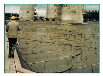
Rebar set into the roof structure keep the PROVOTON foam concrete impact layer connected to the platform.
