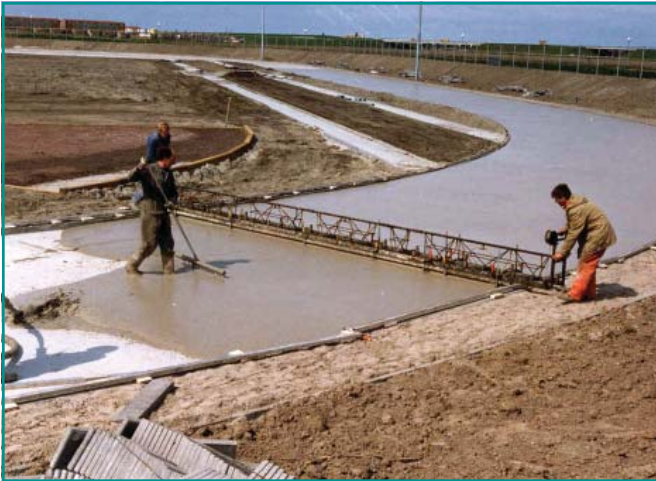
The final lift of foam concrete being leveled during placement.
